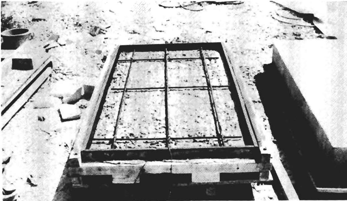
**Figure 1. First Stage Construction of Panel with LMC Overlay.**
