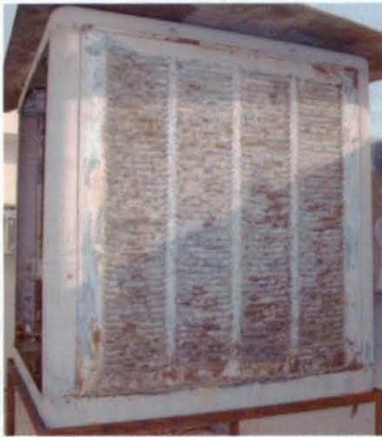
Fig. 2. The effect of the cumulated salt on the evaporative cooler (outside the cooler).
