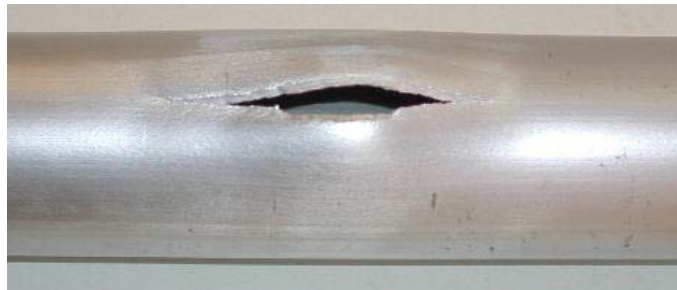
Fig. 15b: The rupture in the aluminum pipe after its bulging.
