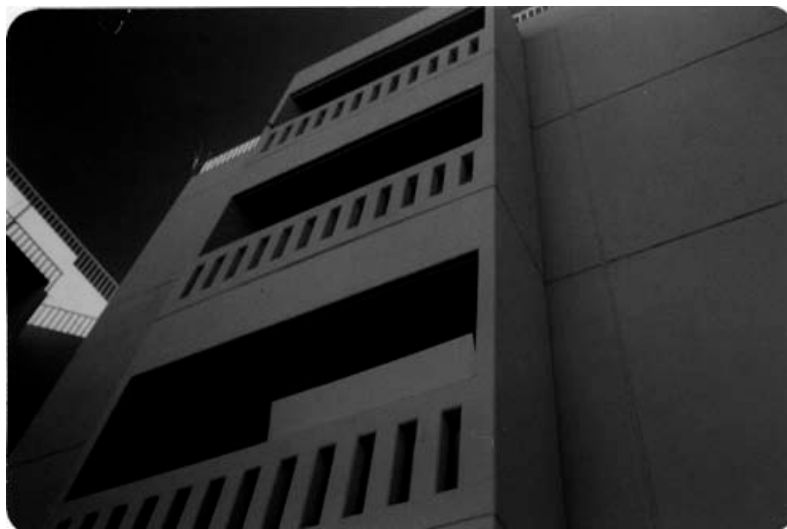
Fig. 11. Utilizing upper part of balcony for more storage.
